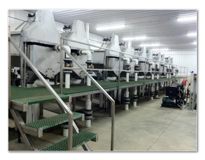
Reliable, self cleaning DTE360 separators have the versatility for multiple applications within stormwater and wastewater management.
